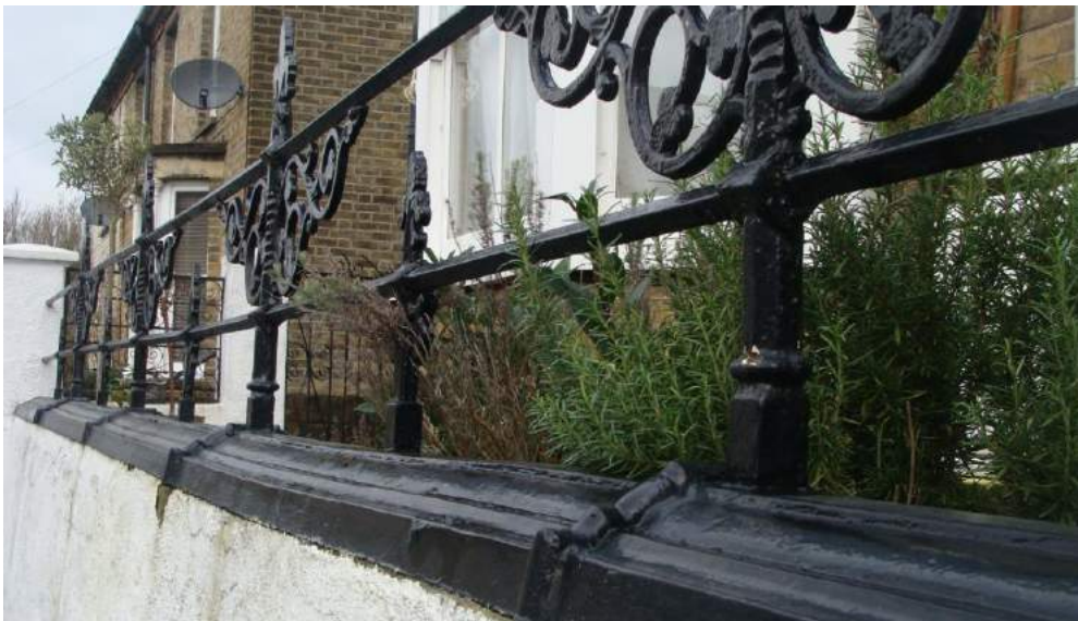
Picture 84. Very good quality early 20th century railings that are protected and which should be retained.
