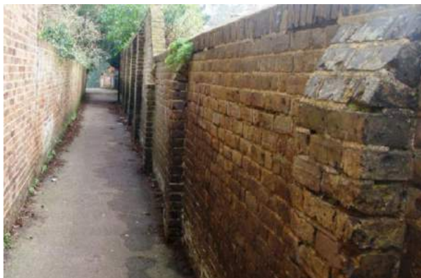
Picture 85. Walls enclosing public footpath 85.
