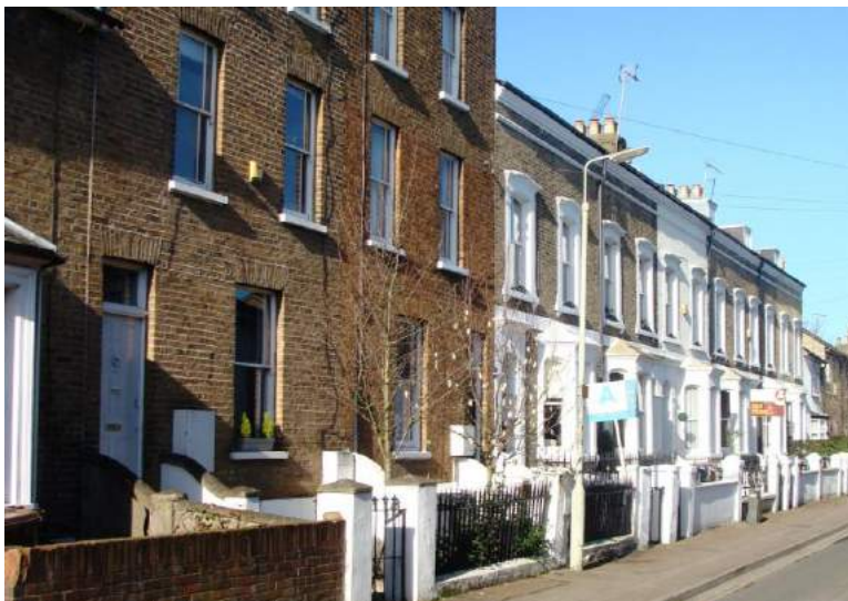
Picture 164. West side of Villiers Street, an attractive grouping with a wide range of good quality detailing most worthy of retention and preservation.
