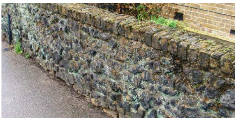
Picture 176. Unusual clinker wall construction to front of properties on Tamworth Road, worthy of retention and additional protection.
