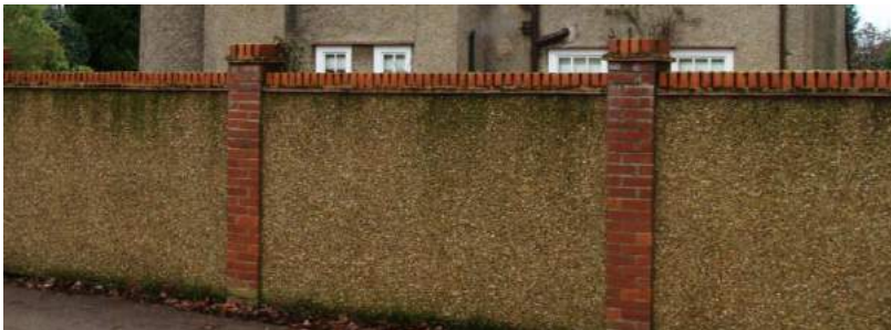
Picture 80. Unusual 20th century wall detailing to Wisteria Place.
