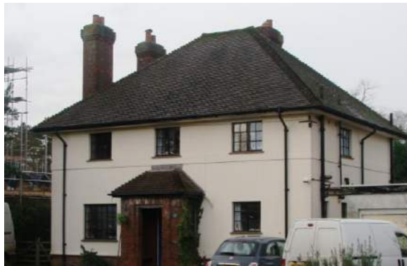
Picture 60. No. 17 Bengoe Street. Some mid/late 20th century properties representative of their age add interest and diversity to the street scene.
