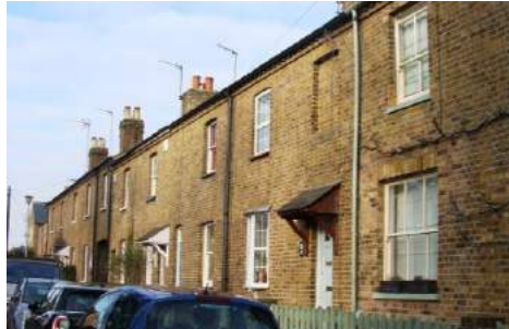
Picture 73. Balfour Street a typical 19th century street with some early porch detailing still remaining. Wouldn't it be nice to carefully replicate this detail above other entrances?
