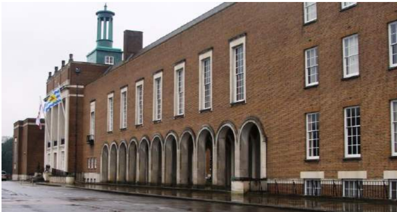
Picture 149. County Hall Architects James and Bywaters and Rowland Pierce. Design influenced by Swedish Romantic and Neo-classical architecture of the earlier 20th century and the work of Sir John Soane.
