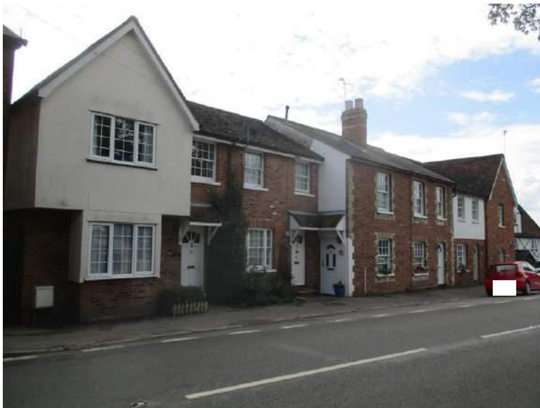
8c and 8d Green End. An example of a good historic building now extended. Of good form, but note the use of poor quality doors and windows
