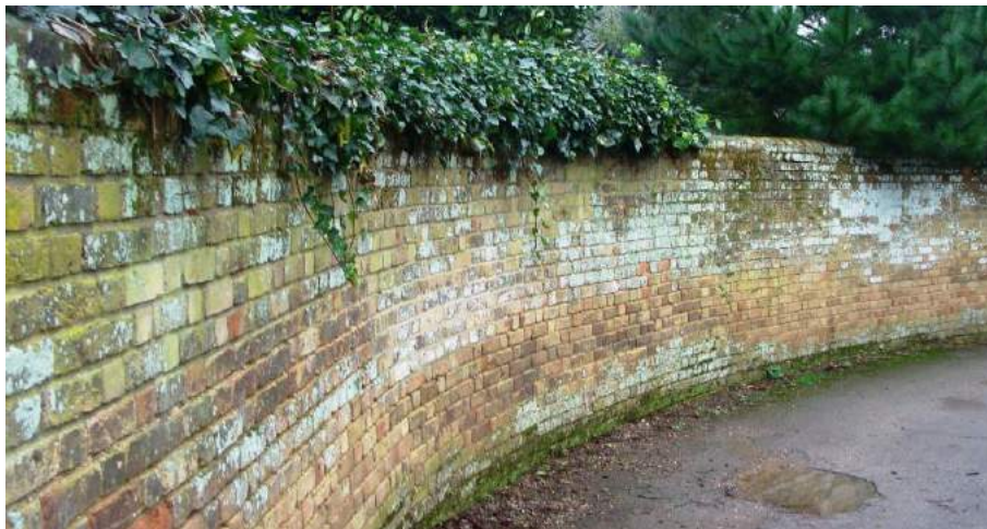
Picture 112. Attractive curved brick wall to Revels Hall. Adds to the quality of the street scene near St. Leonard's church.
