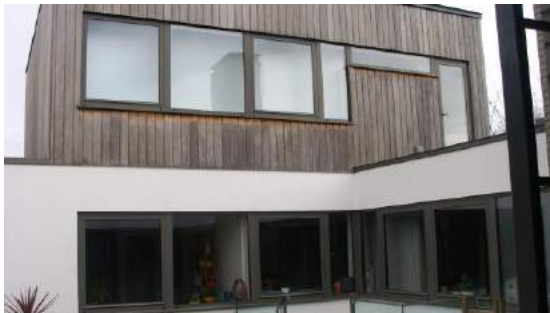
Picture 143. Hide House Railway Place. Hide House 2B Railway Place. A modern 'eco' solution. The owner advises this house is super insulated with some green roof space. Solar panels, air source heat pump system, heat recovery system and controlled lighting. John Pratley, Building Futures Awards Judge, said: "Hide House is an interesting attempt to construct a low energy home at a reasonable cost. The owners have created a house which makes excellent use of daylight and provides very good use of the available land on a very constrained site. The owners should be congratulated for designing and building a very attractive home on a very difficult to exploit site."
