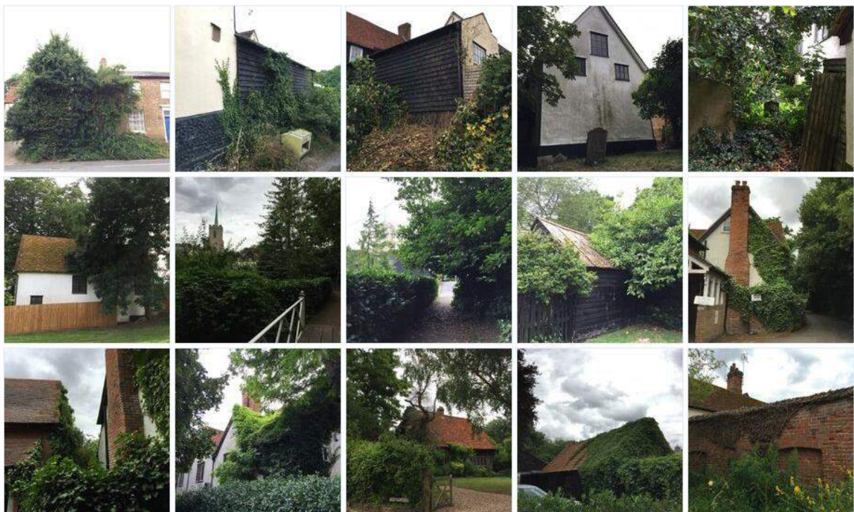
Overgrowth of vegetation
