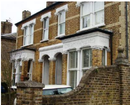
Picture 167. Decorative detailing to Nos. 51-53 Ware Road. Note boundary wall worthy of retention.
