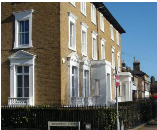
Picture 168. Very fine unspoilt building corner of Ware Road and Townshend Street that makes a most imposing presence in this part of the conservation area.
