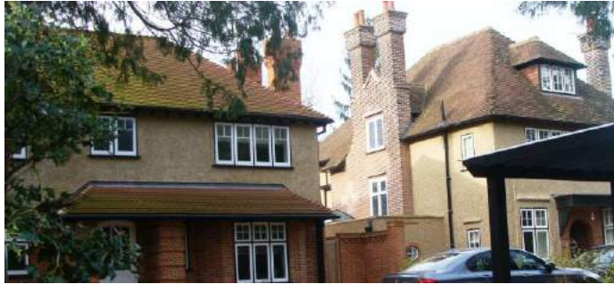
Picture 130. Quality 20th century housing on Morgans Road, note impressive chimney detail.
