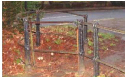
Picture 142. Boundary railing detail and entrance point to All Saints churchyard, south western corner.
