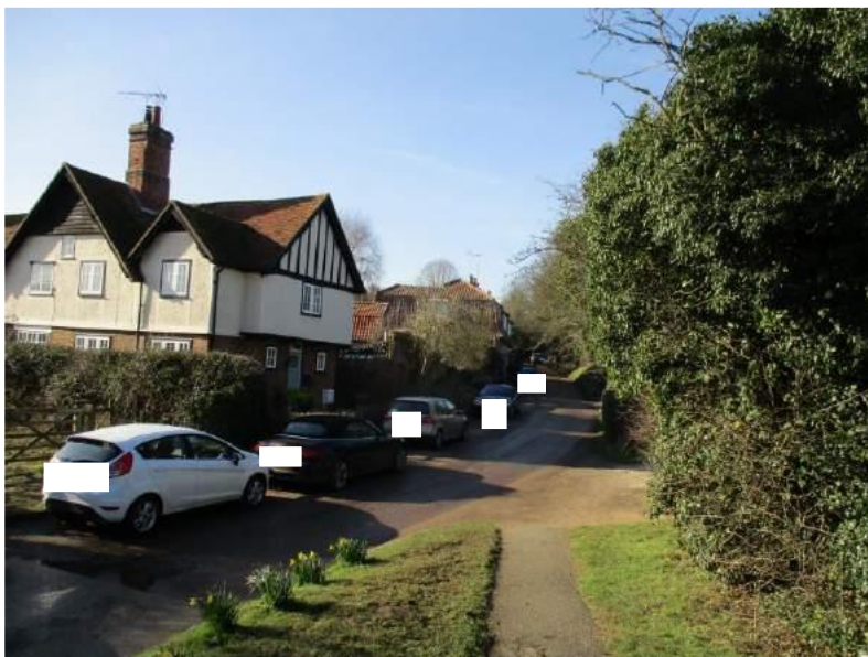
3 Malting Lane and wall with No. 2. Category 1.
