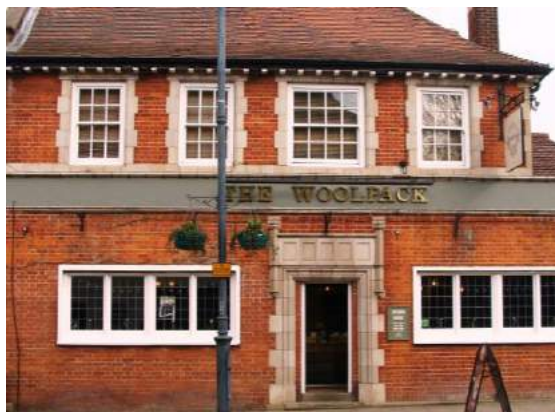
Picture 321. The Woolpack PH nicely proportioned and detailed commercial building.
