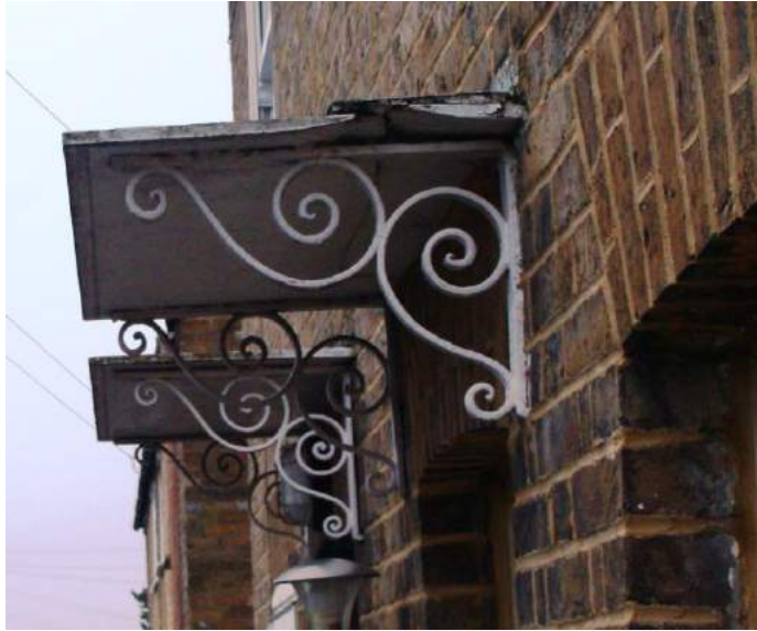
Picture 104. Early canopies on metal bracket supports which add to the interest of the street scene and which are worthy of retention.
