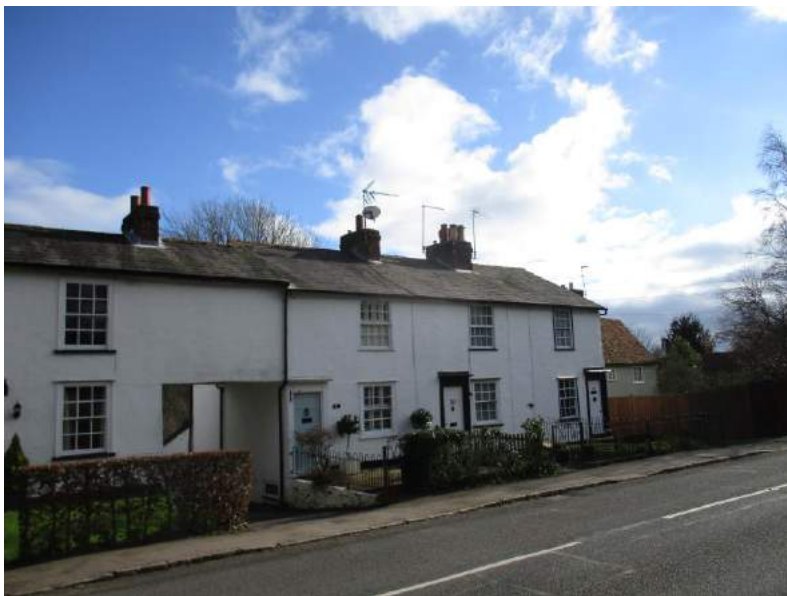
Good quality boundaries to Nos. 36-44 (even) Green End. Note the contrast to the south.
